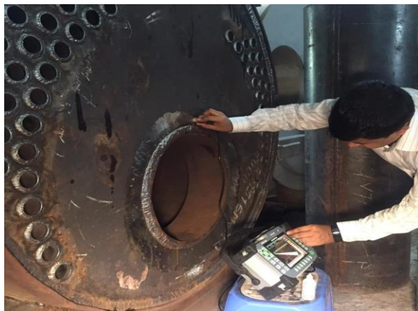
Boiler Manufacturing Stage Inspection (Ultrasonic Flow Detection Test)
